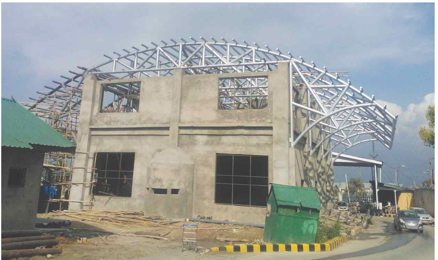
▲ Shrinagar International Air Port - 125 M.T.
